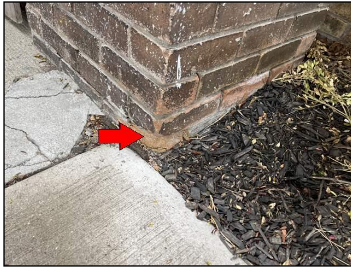
6. Spalling
