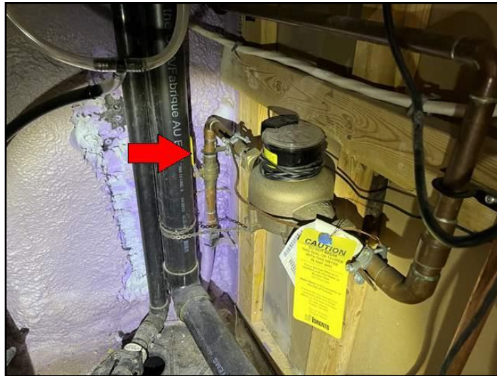
15. Main water shut off valve
