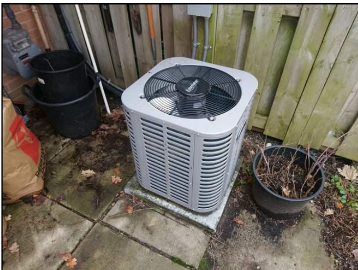
Air cooled condenser
