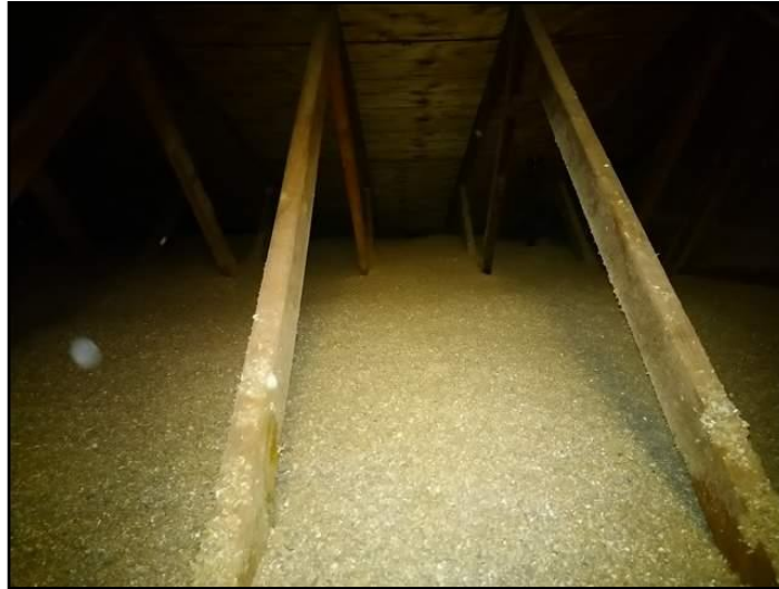
Cellulose over fibreglass
