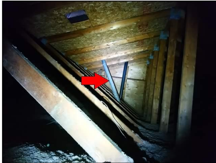
Exhaust duct not insulated in attic
