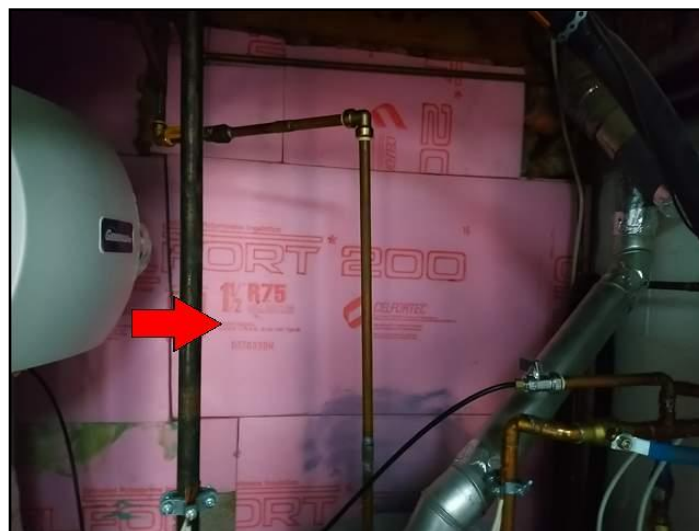
Ex: Exposed foam insulation
