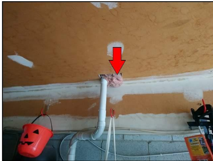
Ex: Unsealed opening in garage ceiling
