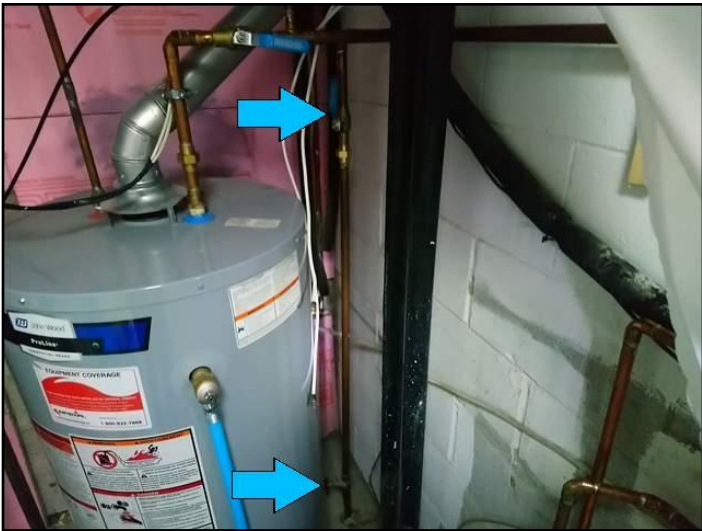
Main water shutoff valve(s)
