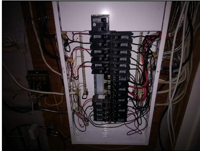
Breaker panel (cover removed for inspection)
