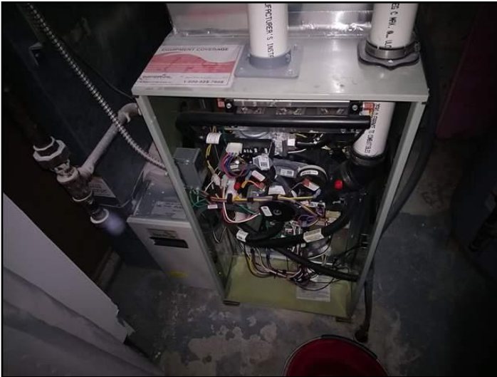
High-efficiency gas furnace
