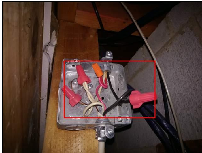
Connectors not compatible with aluminum
